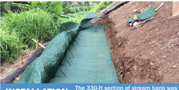
INSTALLATION The 330-ft section of stream bank was reinforced and stabilized with a 8-ft high PYRAWALL
