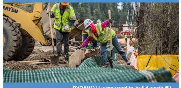
INSTALLATION PYRAWALL was used to build earth-fill embankment approaches
